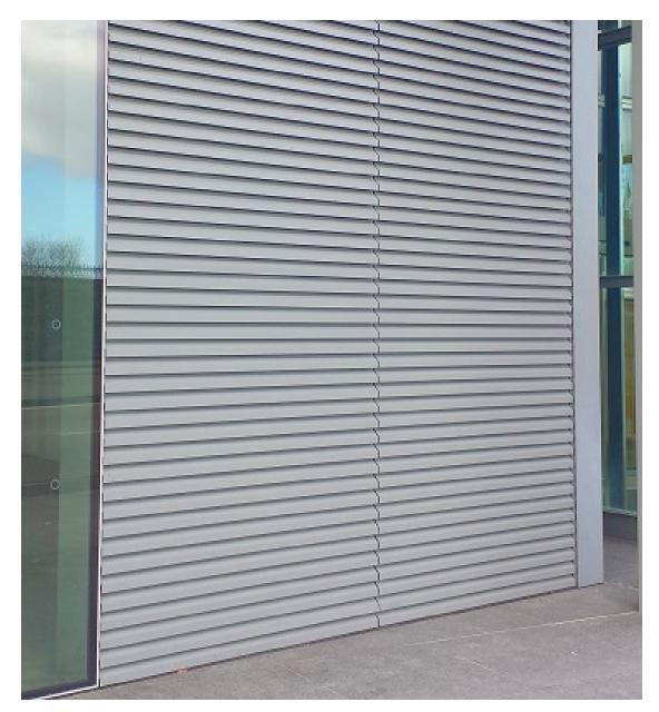
Single bank extruded aluminium louvre pitched at 75mm with a 35mm front face. A bespoke design to achieve the architectural design intent. The system achieved Class A4 up to 0.5m/s and Class B4 up to 1.0m/s face velocity.
