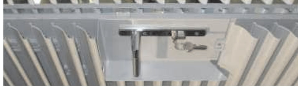
Front view and locking detail of one of the 3100mm wide x 2650mm high double doors featured above.
